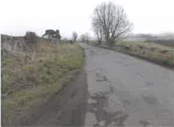
Access track at junction with B7060 and rightwards visibility
